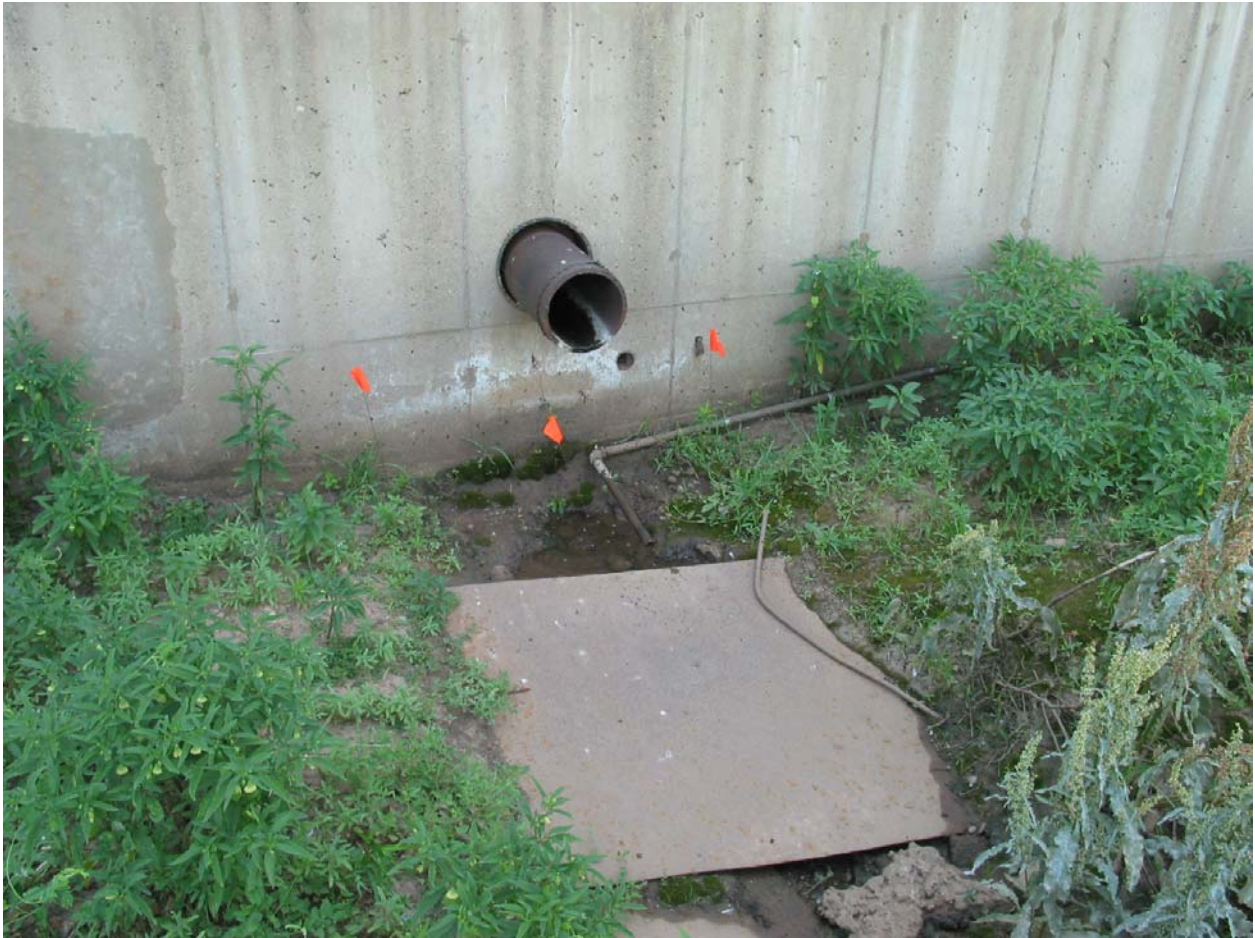
Figure 2 - Drainpipe Location With Flagged Sample Locations
